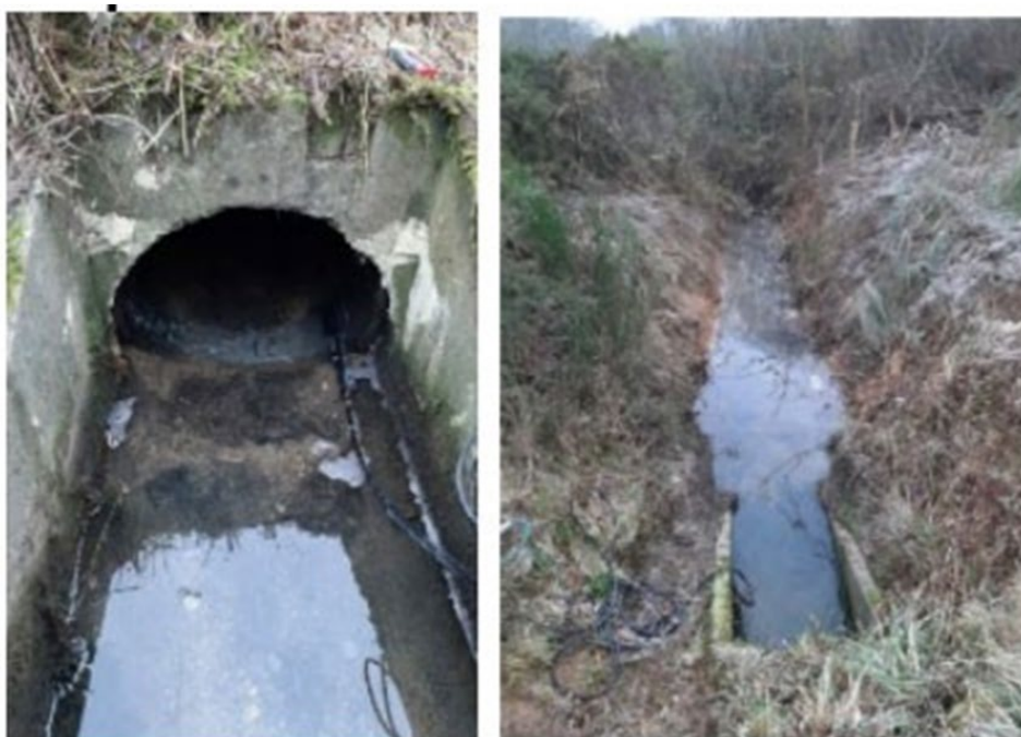
FIGURE 5 – EXUTOIRE DU BV4 DN600
