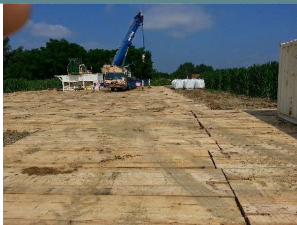
FIGURE 52 – PHOTO DE PLATELAGE
